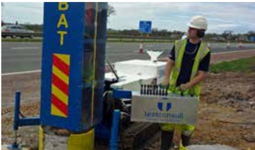
**Our high strain dynamic pile testing offers a fast and cost-effective method of determining the performance of pile foundations.**
