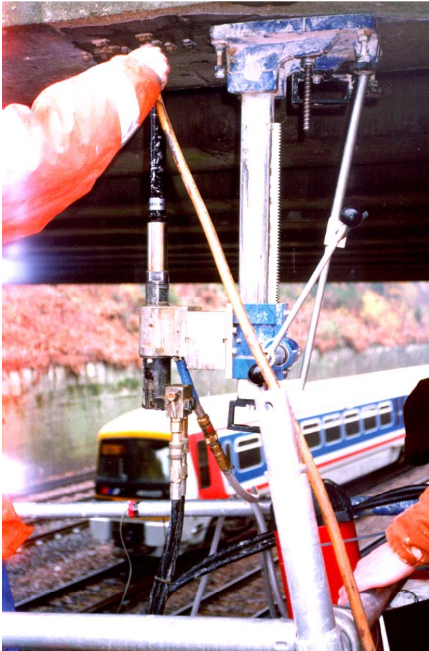
Photo above – Measurements are taken on vibrating wire strain gauges at each increment of core drilling.
